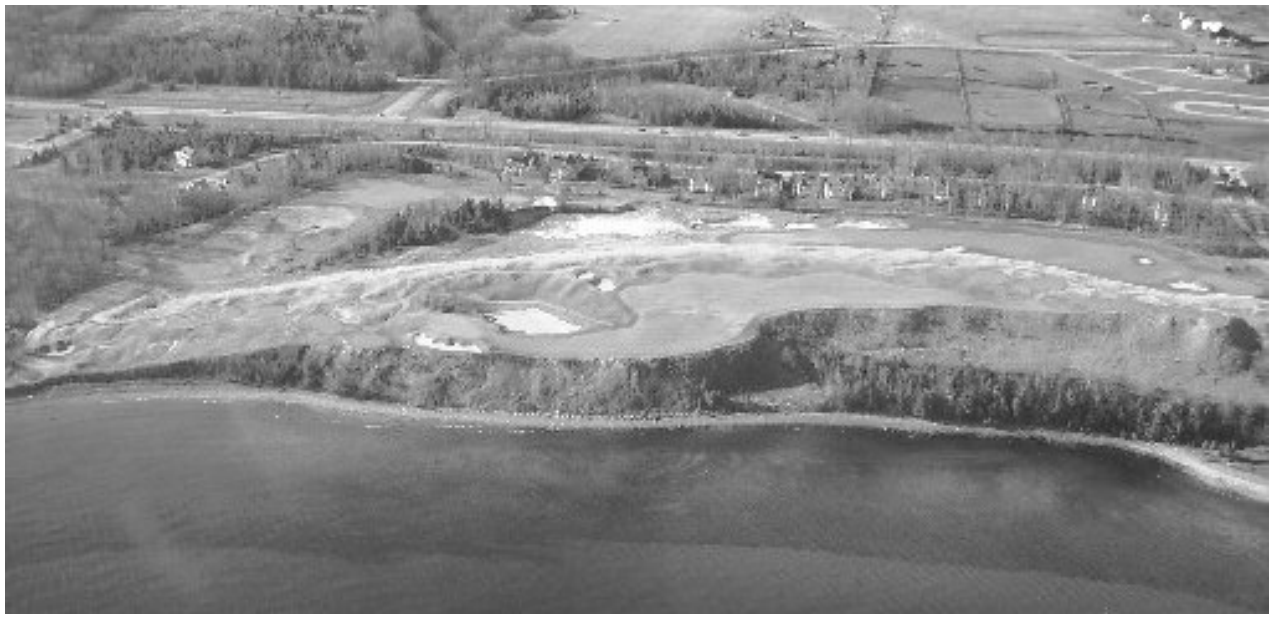
Aerial view of Bay Harbor shoreline when the effects of CKD leachate were visible. COURTESY PHOTO
